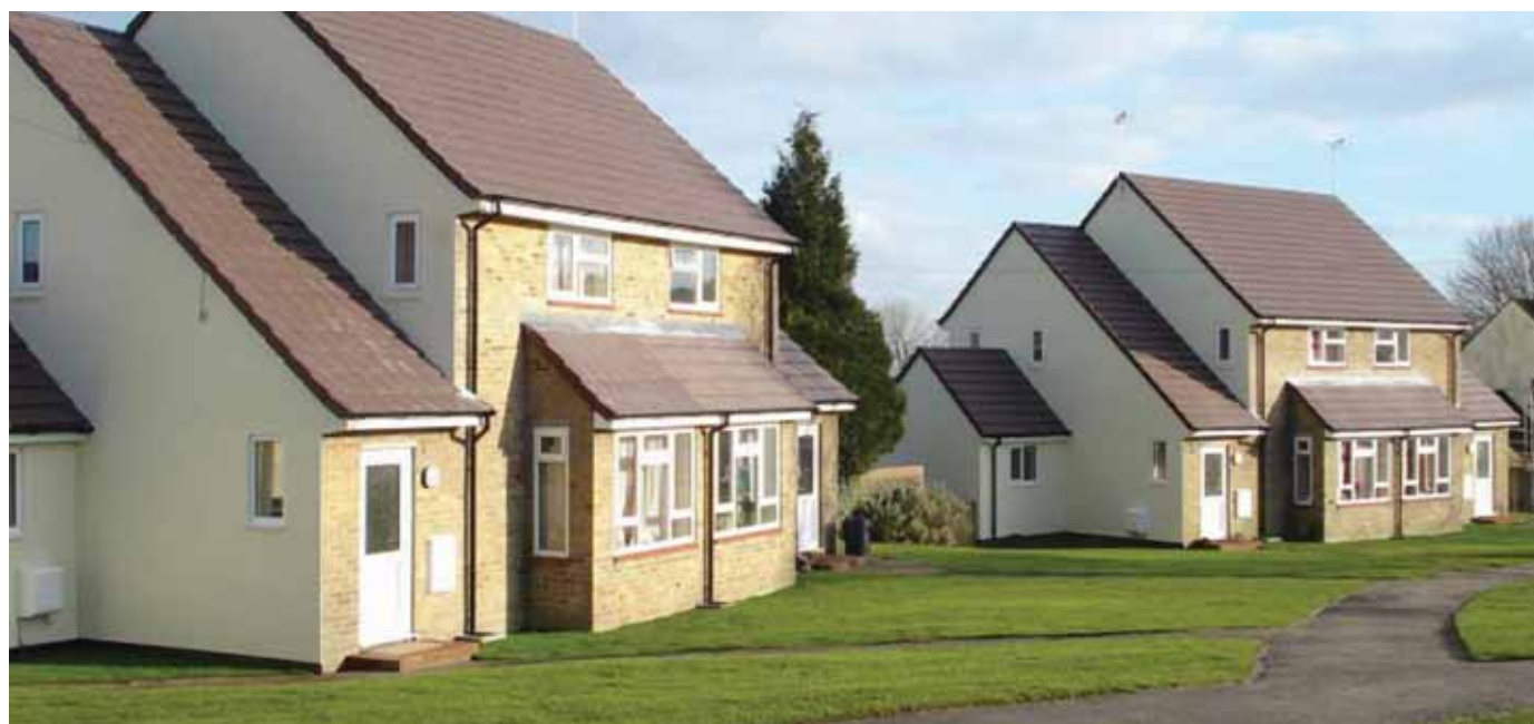
Modern Service Family Accommodation (SFA) at Blandford Camp in Dorset
